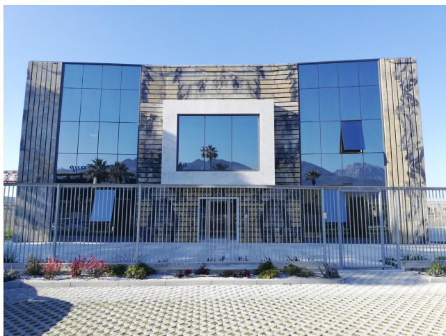
SLABS WAREHOUSE IN ITALY DEPOSITO LASTRE IN ITALIA
